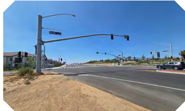
Figure 5. Missing Sidewalk near Alessandro Boulevard and Darwin Drive
